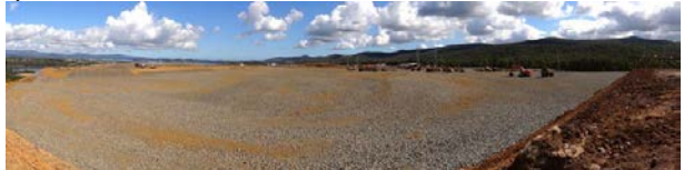
Completed pulp mill platform one
