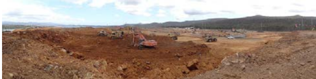
Early work on the pulp mill platform one
